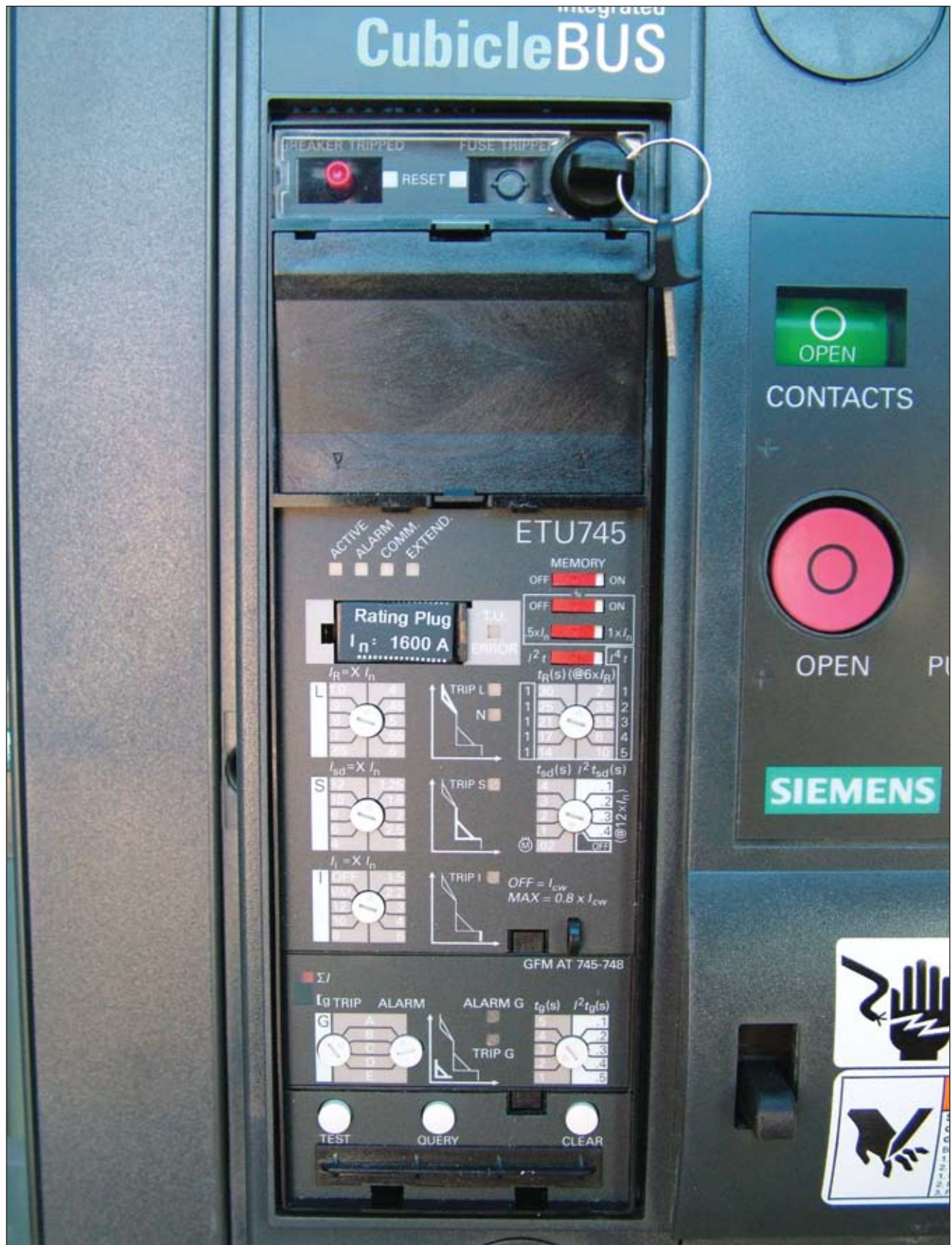
Photo 4. Main circuit breaker trip unit
