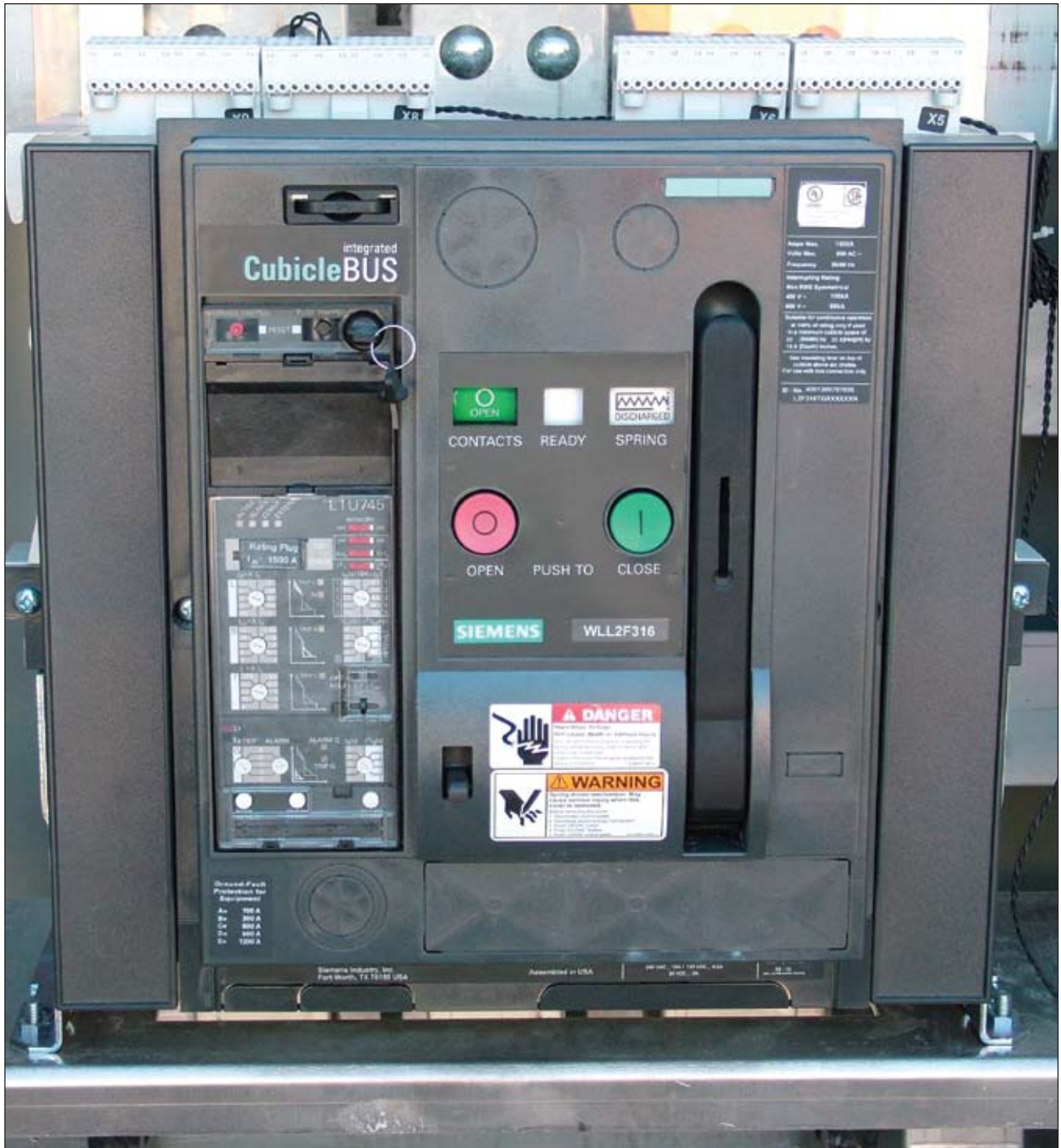
Photo 3. Main circuit breaker with ground fault
